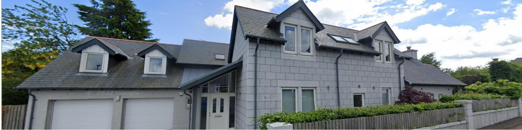
5 Kirk Drive (formerly 22 Kirk Crescent South)
