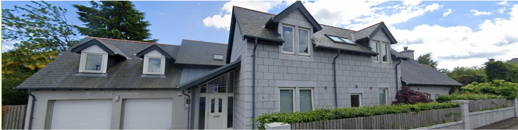
5 Kirk Drive (formerly 22 Kirk Crescent South)
