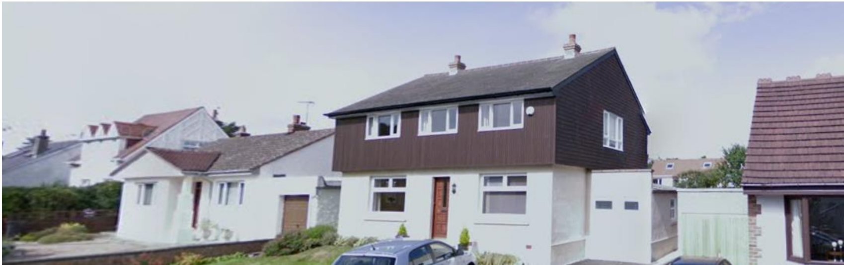
11 Kirk Crescent South – original house (note significant change in footprint in terms of how far back the property extends)
