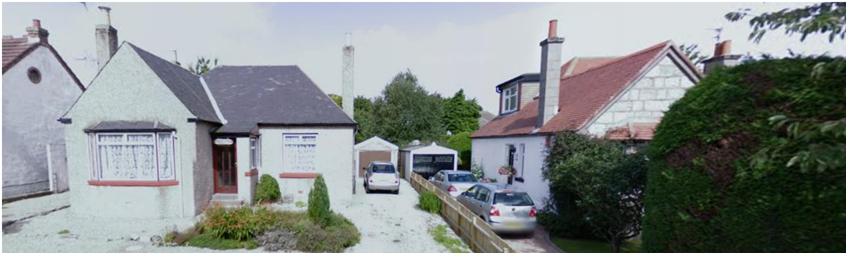
15 Kirk Crescent South – original house (note the significant change in both height and footprint)
